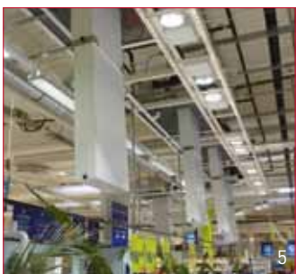
Chutes for direct filling of supermarket displays with flake ice
